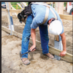
Attach Splash Board
